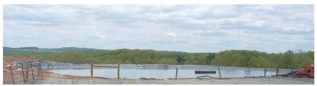
Photo 5.20 c Fresh water supply pond. Black pipe in pond is a float to keep suction away from pond bottom liner. Ponds are completely enclosed by wire fence. Source: NYS DEC 2009.
